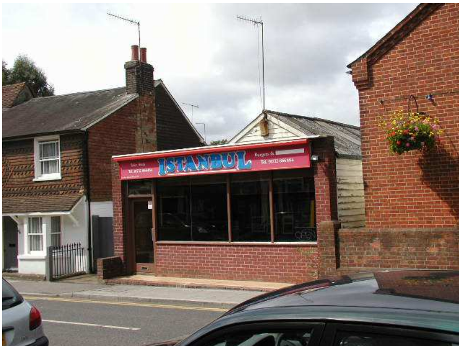
39 Unfortunate shopfront adjoining listed building
