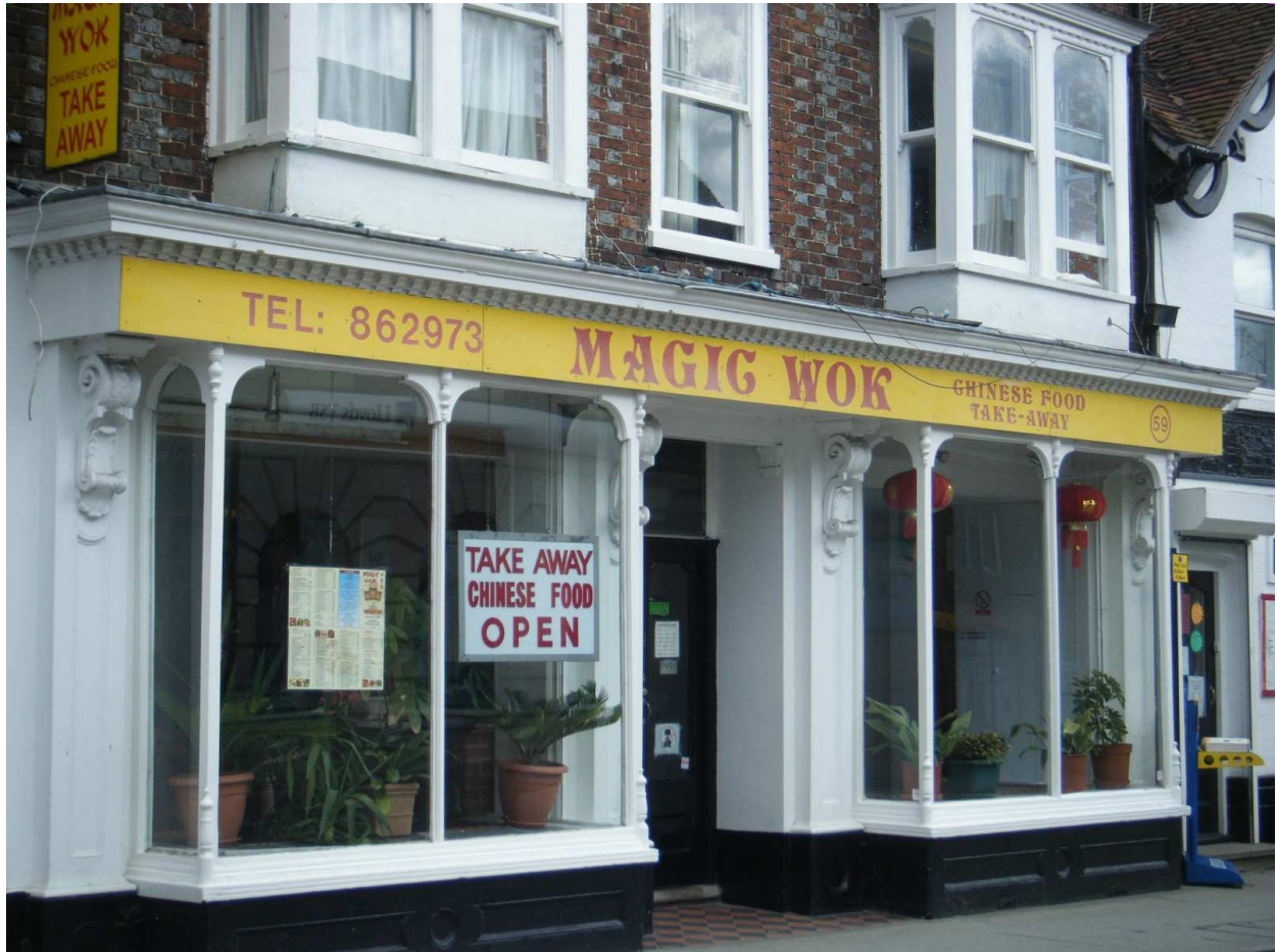
49. Another attractive shopfront in the High Street
