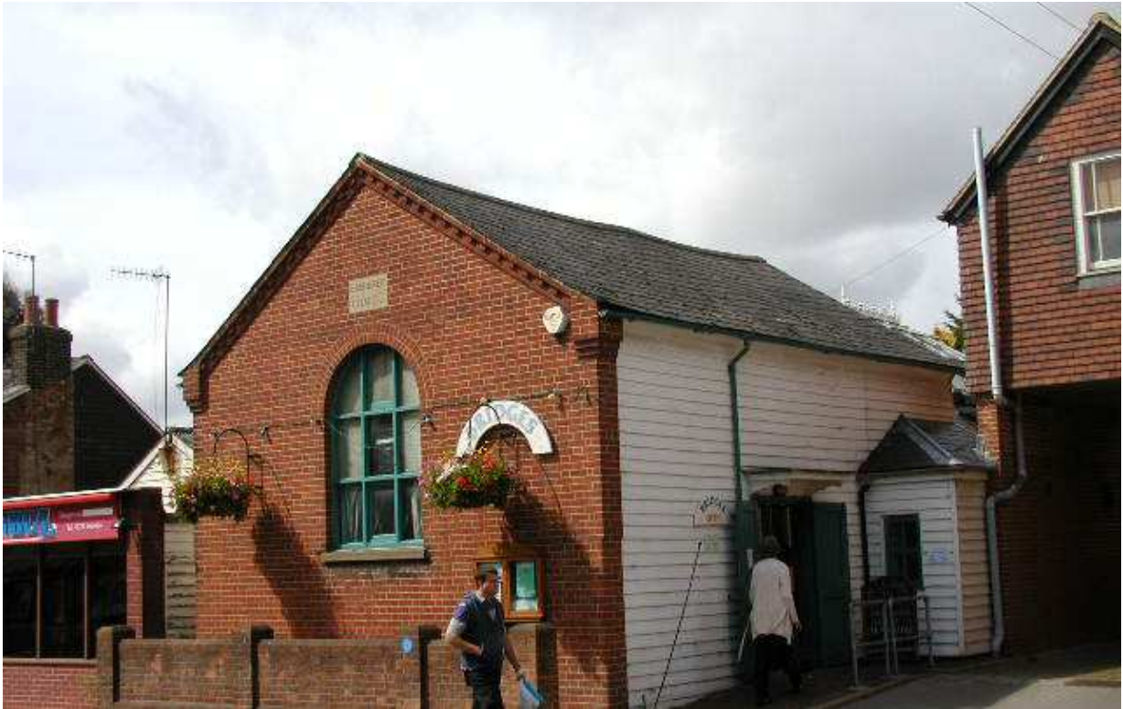
2. Historic ~Listed Chapel - now a community centre
