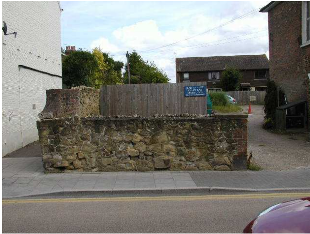
41. Portion of historic wall adjacent to No. 47
